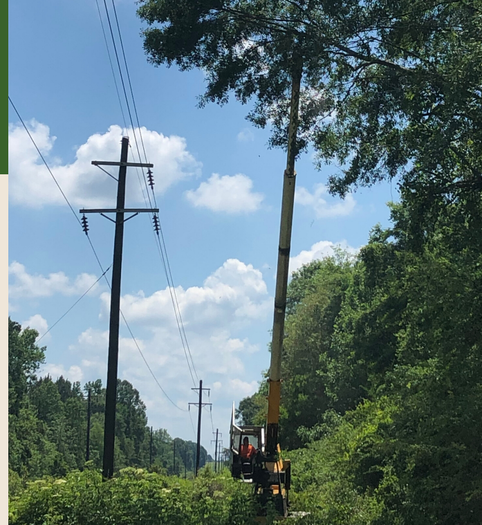
Side trimmer being used to trim tree alongside of Cooperative Energy's right-of-way
