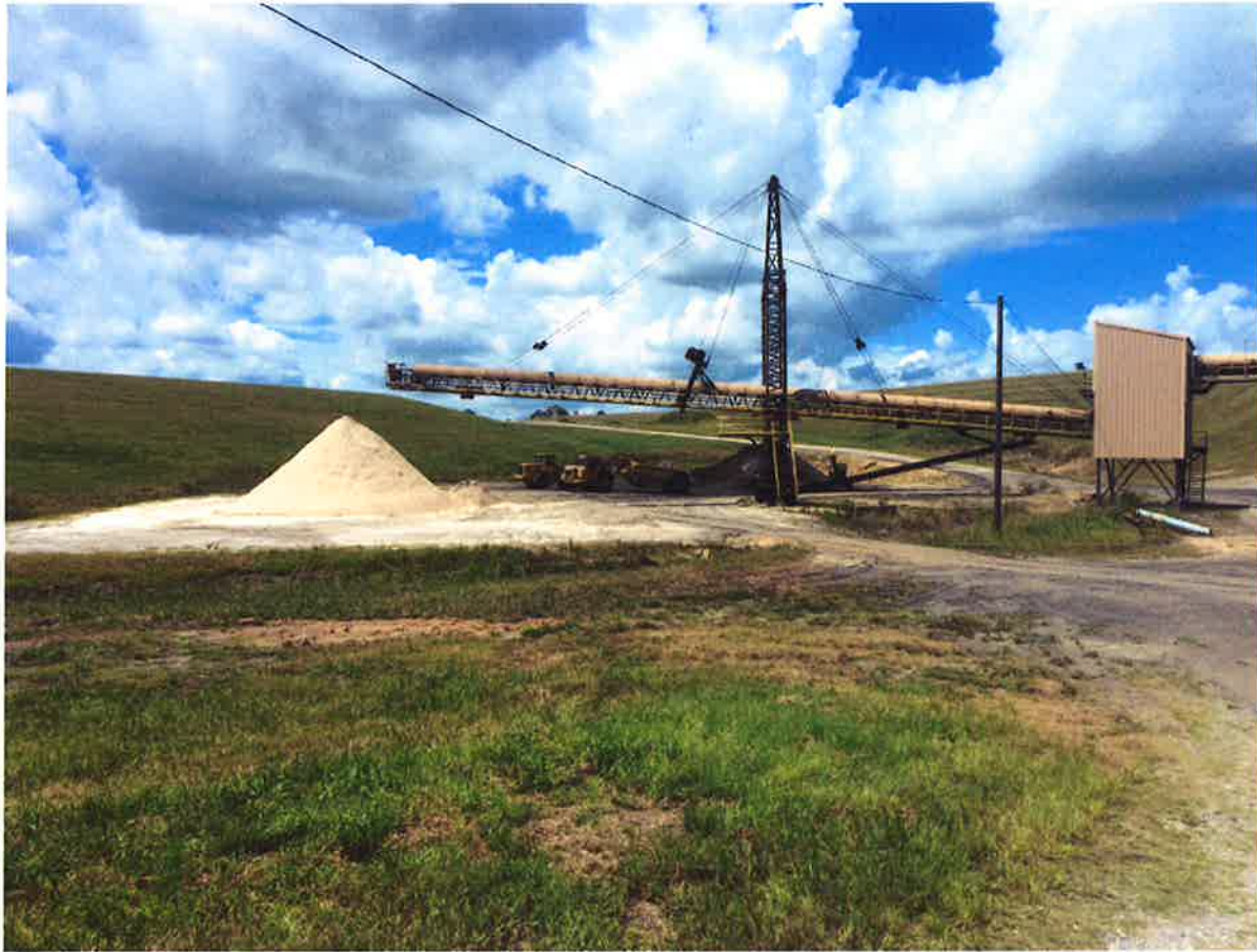
Figure 4-7: Radial Stacker Area
