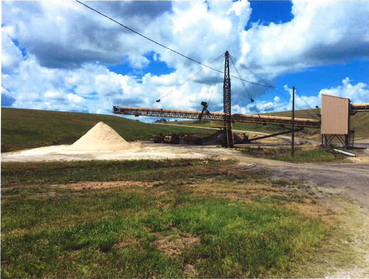
Figure 4-7: Radial Stacker Area
