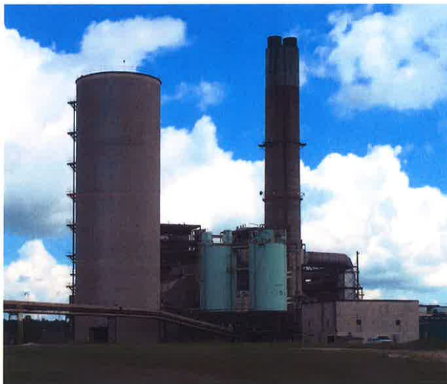
Figure 4-3: Fly Ash Silos and Conveyor to the Landfill
