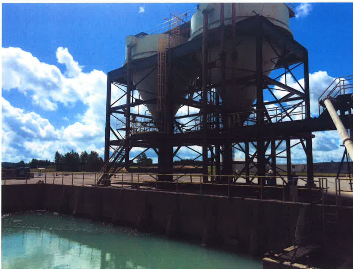
Figure 4-2: Bottom Ash Dewatering Bins and adjacent Settling Surge Basin
