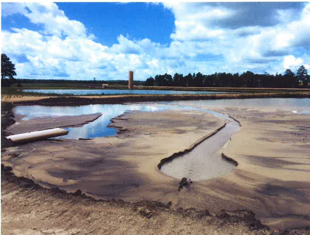
Figure 4-6: Emergency Scrubber Pond (near) and Scrubber Supply Pond (far)
