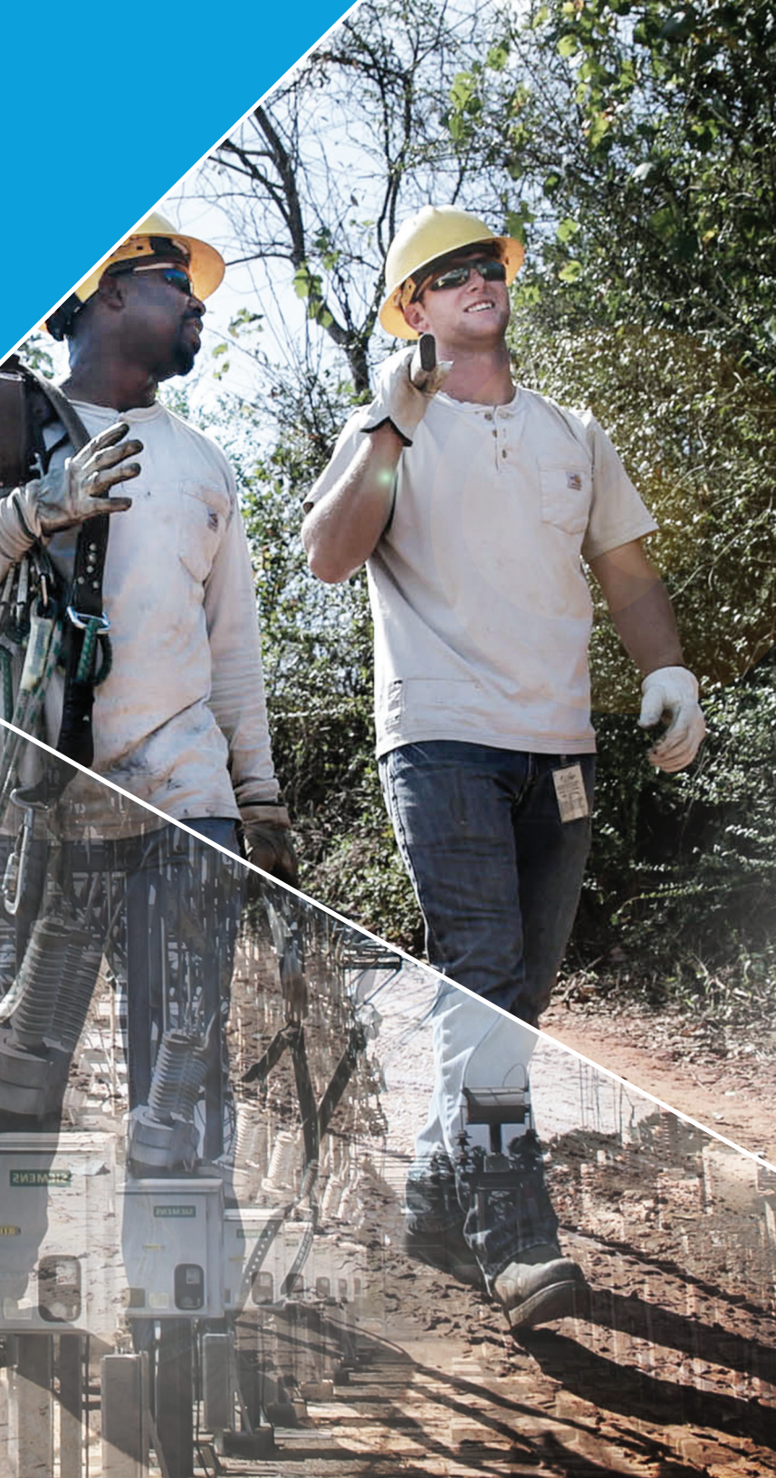
Left: Circuit Breaker at the J.T. Dudley, Sr. Generation Complex Switch Yard Right: Lineman II Michael Bolton (Left) | Lineman II Jared Davis (Right)
